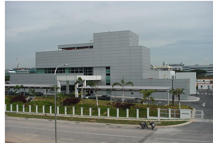
Singapore Avago Manufacturing Site
