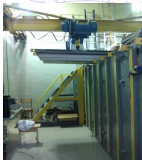
Passive shielding - 60 tons
